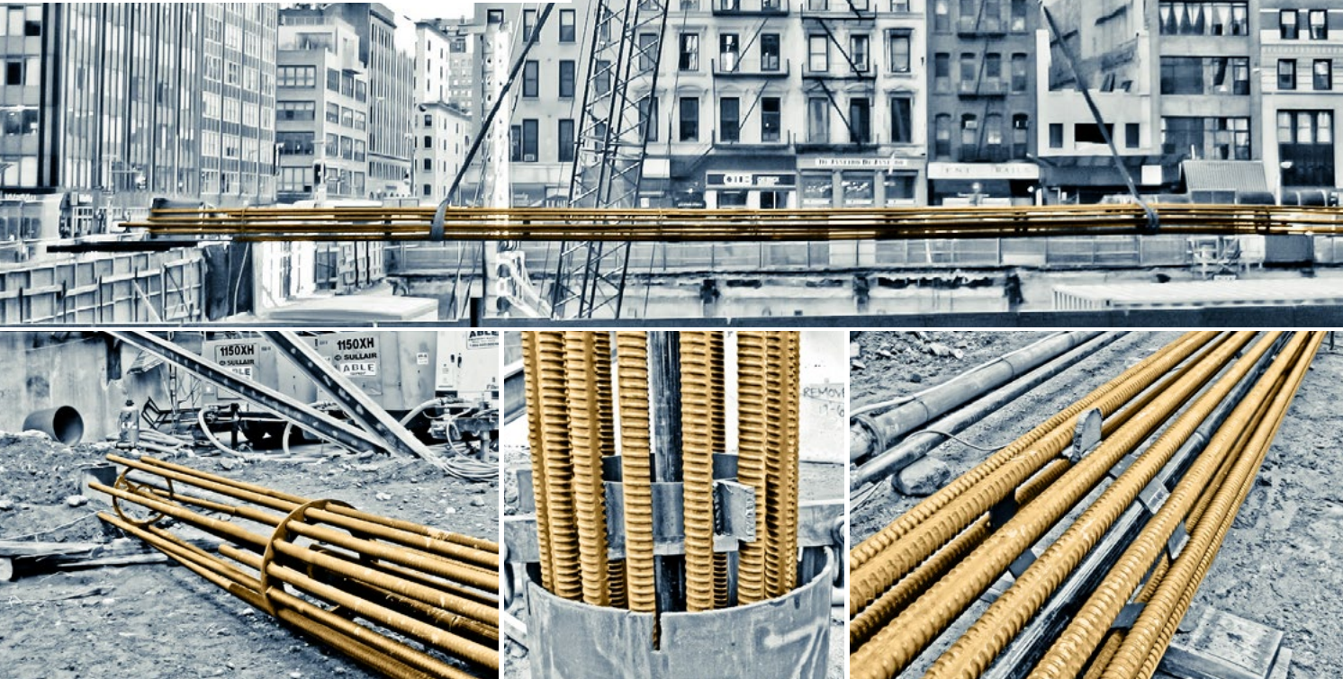
99 Church Street, New York, USA
