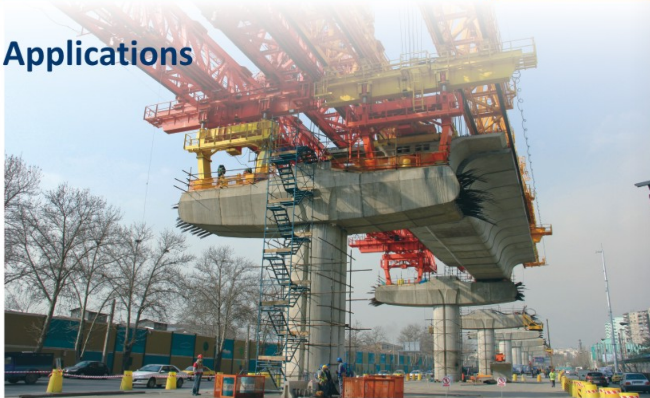
Sadr Bridge, Iran, 2012
